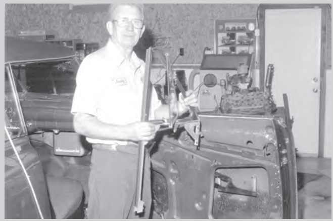
Jim prepares to install the newly restored vent window in door repeating steps from number 6 back to number 1.
