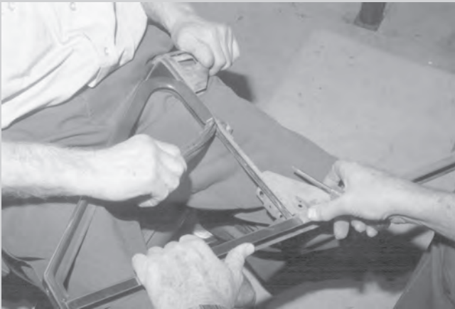
Remove old rubber vent window seal from frame by hand.
